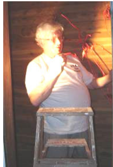
Mike Stroupe made sure all the wires were routed properly
