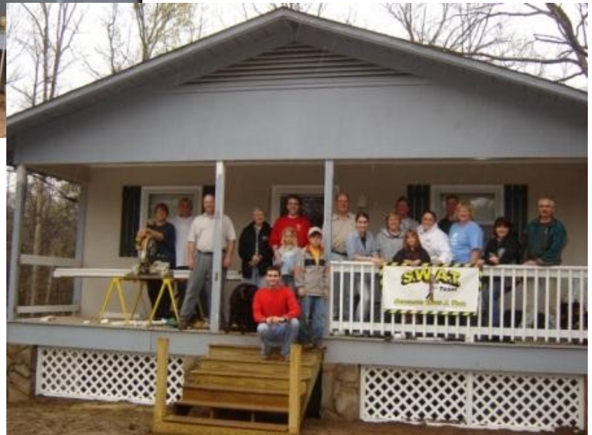
Right: Although the SWAT Team did not finish all the work to be done, their hard work really shows in the "after" picture
